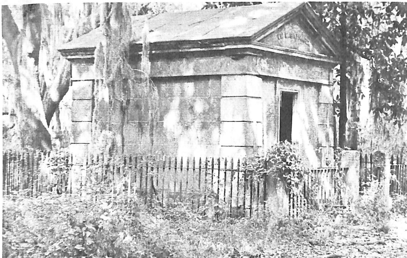
The Baynard Mausoleum served as the collecting point for several generations. It remains, across from the present library site, as the largest intact antebellum structure on the Island.
