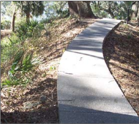
Left: Visitors, especially the elderly, were uneasy on this walkway. Note how it fell off steeply to the left, with part of the walkway tilted in that direction.
