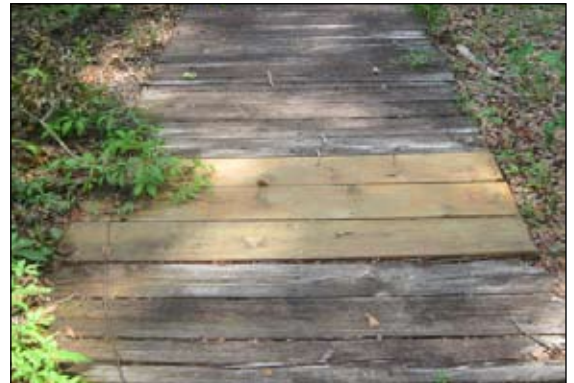
Left: Ladies especially could catch their heels in the rotting planks of this picturesque walkway.
