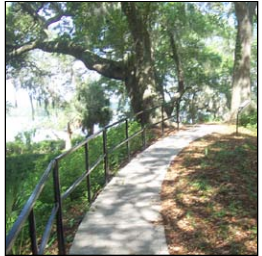
Left: Visitors, especially the elderly, were uneasy on this walkway. Note how it fell off steeply to the left, with part of the walkway tilted in that direction.
