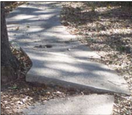
Left: This extreme upthrust of concrete was caused by tree roots and was a stumbling block for any visitor.
