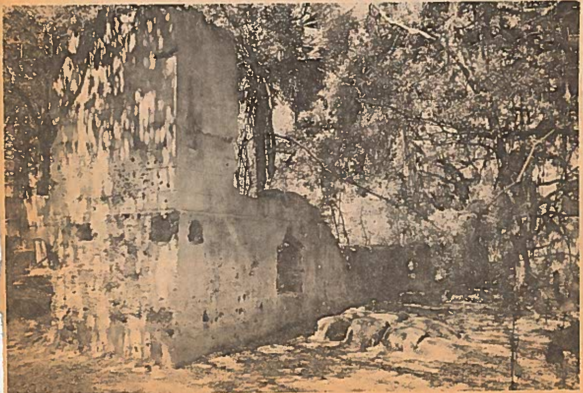
REBUILDING —The remains of William F. Baynard's plantation home in Sea Pines which was built
